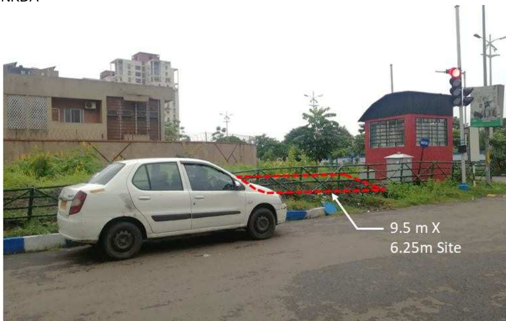
Site 3, Existing Site Photograph
