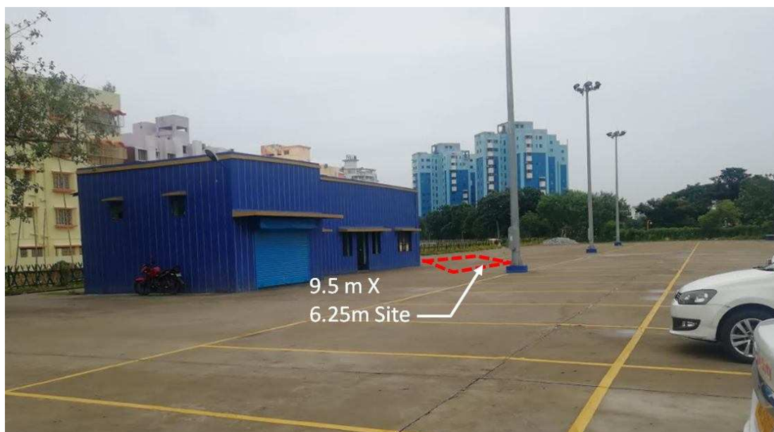
Site 2, Existing Site Photograph
