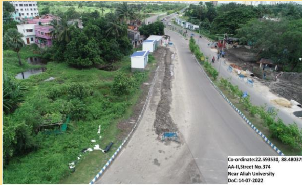
Identified stretch near Alliah University post installation of Gas Pipeline
